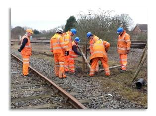
Left – members of the PRNB team installing fence corner post at the rear of the signal box. Care being taken to identify the location of electricity supplies and any other underground installations.
